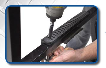
Using the hardware retained from step 1, attach rail assembly to cross member and rail bracket as shown.
