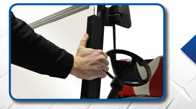
Attach windshield to cart by snapping strut brackets to front struts.
